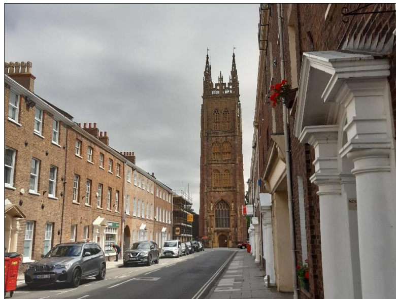
Photograph 21: View along Hammet Street towards the Grade I Church of St Mary Magdalene
