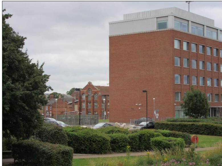
Photograph 18: Grade II Listed Barnicotts, viewed from the north-east from within the Site
