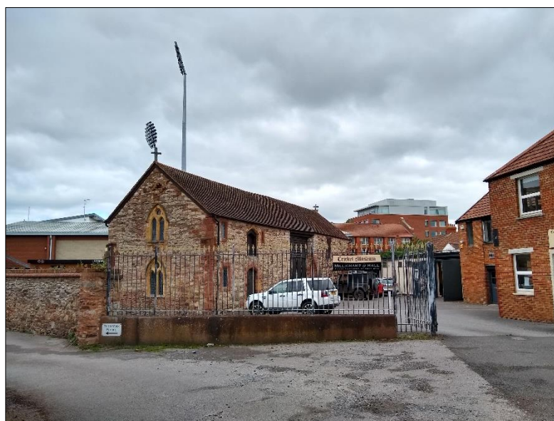
Photograph 11: Grade II* Priory Barn, viewed from the south
