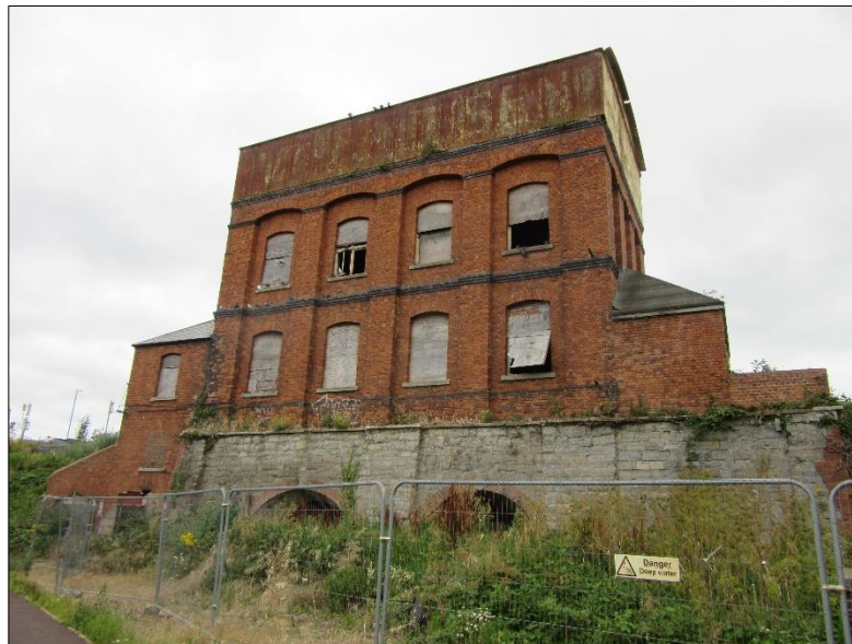
Photograph 13: Grade II Firepool Pumping Station, viewed from the south-east
