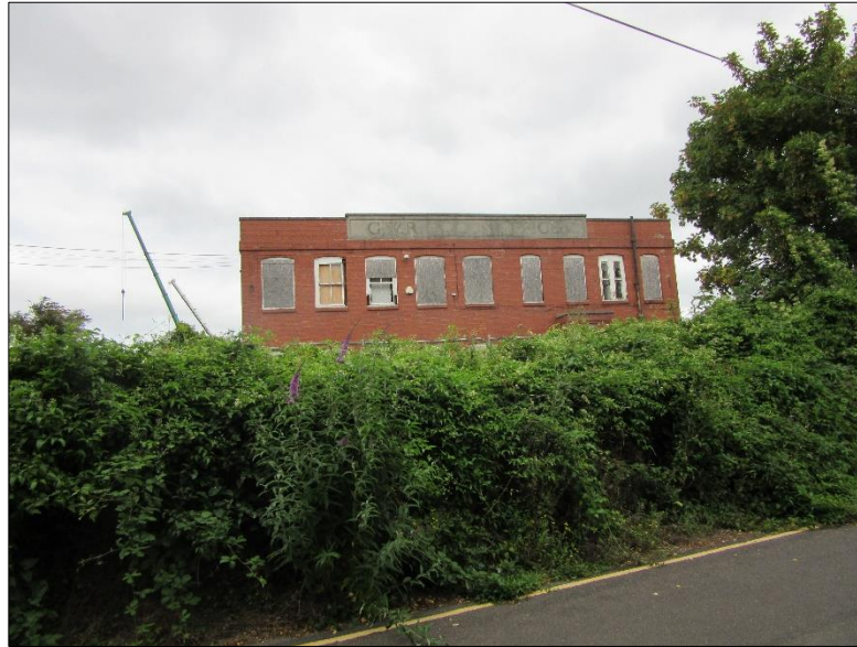
Photograph 7: Former GWR Goods Depot in north of Site, viewed from the south
