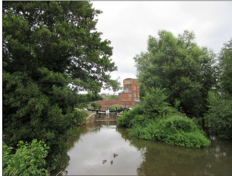
Photograph 15: Grade II Firepool Pumping Station, viewed from the footpath at the eastern edge of the Site
