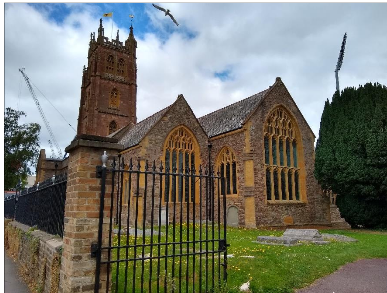
Photograph 9: Grade II* Listed Church of St James, viewed from the east
